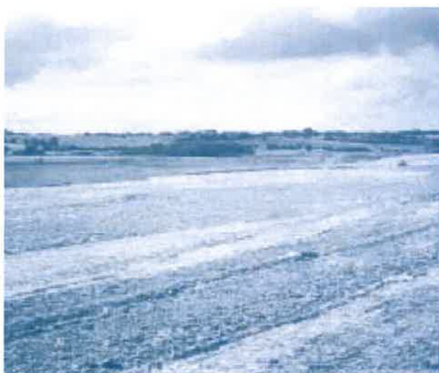
Figure 5.1 | Temporarily capped zone of a landfill
